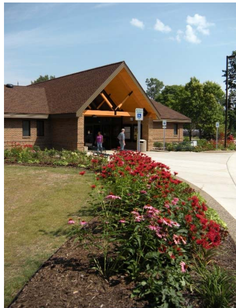
The Swartz Creek Rest Area project was managed and designed by the Roadside Development Unit. This rest area, which was reconstructed in 2008, accommodates 650,000 visitors annually and is also used by the Michigan State Police as a mobile commercial vehicle enforcement facility.
